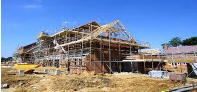
Figure 3.14 Layout causes in construction site
