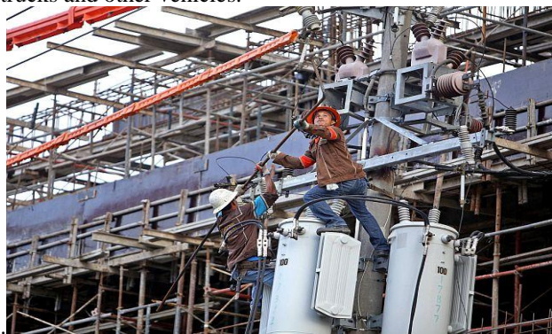
Figure 3.3 electrocutions in construction site
