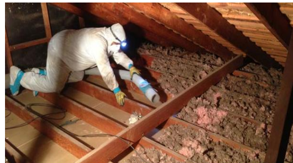
Figure 3.11 Ventilation causes in construction site
