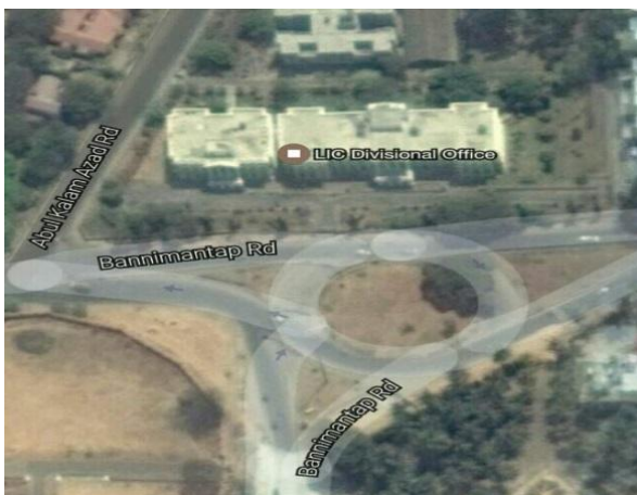
Figure. 3. Improper islands at LIC junction
