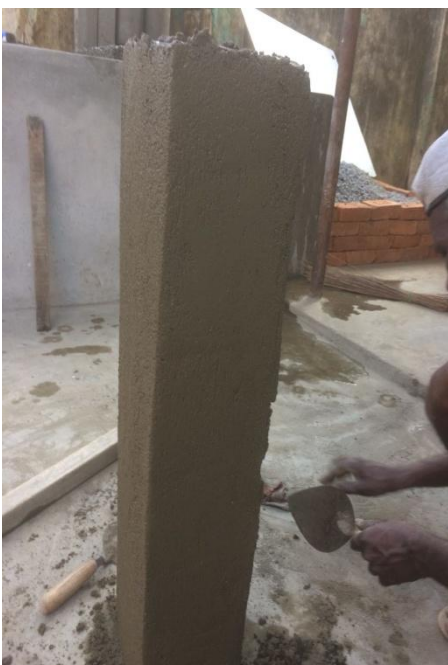
Figure.6. Casting Work Of Scrim Reinforced Column
