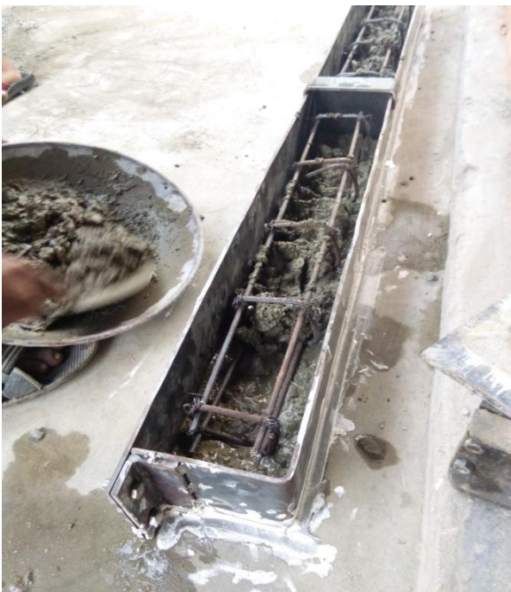
Figure.2. Reinforcement Details
