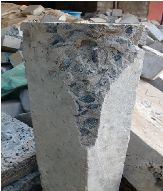
Figure.4. Failure of Conventional Column
