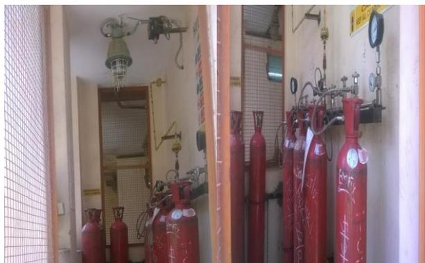
Figure 9.1 Safety Measures for Hydrogen Gas Cylinder
