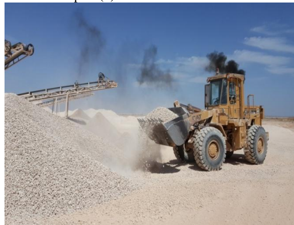
Shovel taking samples from stockpile of coarse aggregates
