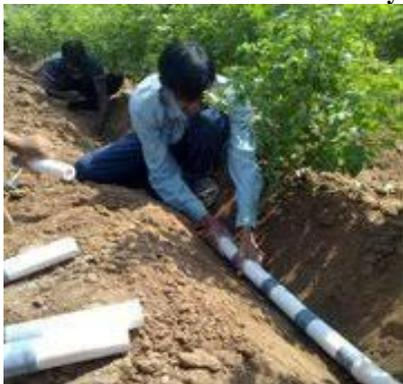
**Figure.4.1 Installation of Porous Clay Pipe**
