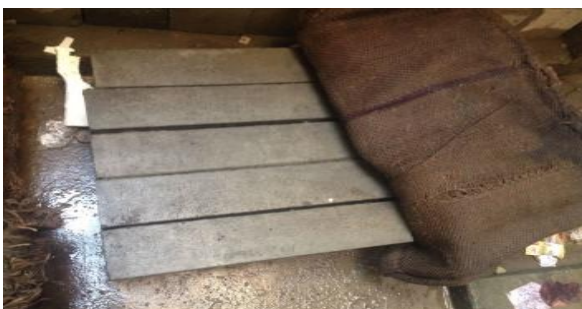
Figure.2. Concrete beam curing
