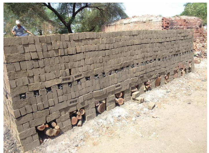
Figure.2. Making of the traditional brick kiln at site
