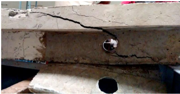
Figure.17. Frame type of failure of Strengthened Beam
