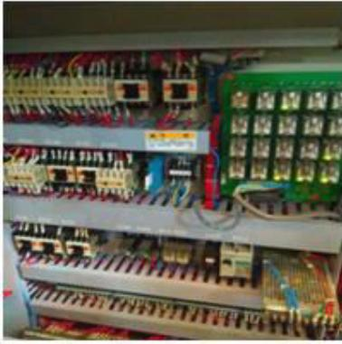
**Figure.1.Pilz Safety Relay**
