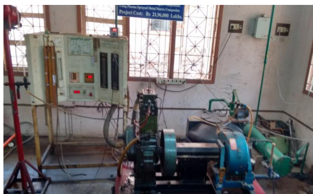
Figure 6.1 Specification of VCR research engine
