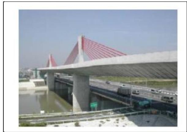
**Figure.4. Shin Meisei Bridge(prospective view) (3-span continuous extra dosed PC bridge)**
