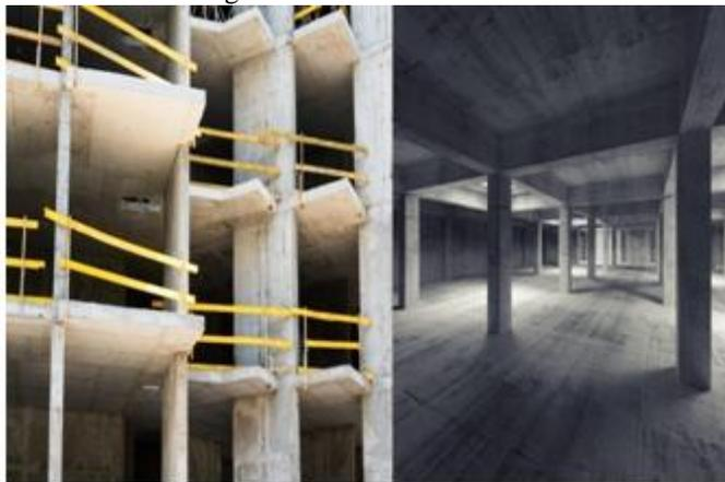
Figure.1. Flat and Conventional Slab Systems
