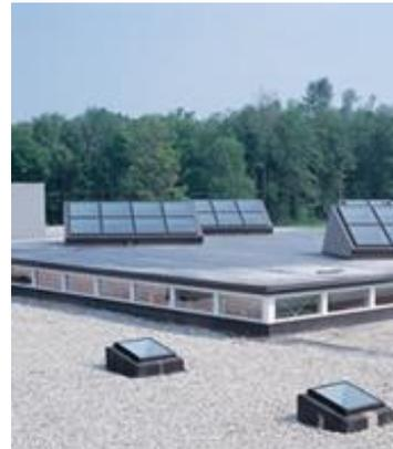
**Figure 2. Roof monitors in commercial building**
