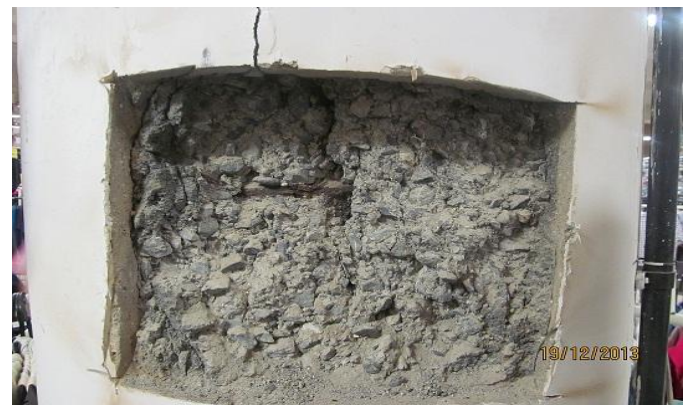
Figure.1. Photograph showing an internal surface of concrete
