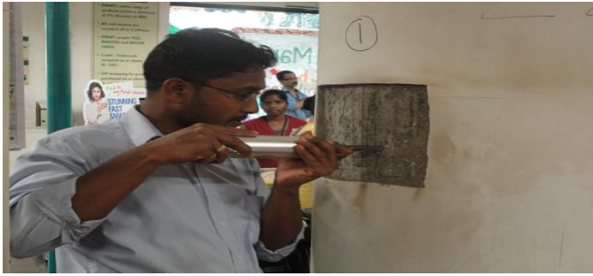
Figure.2. Rebound Hammer test
