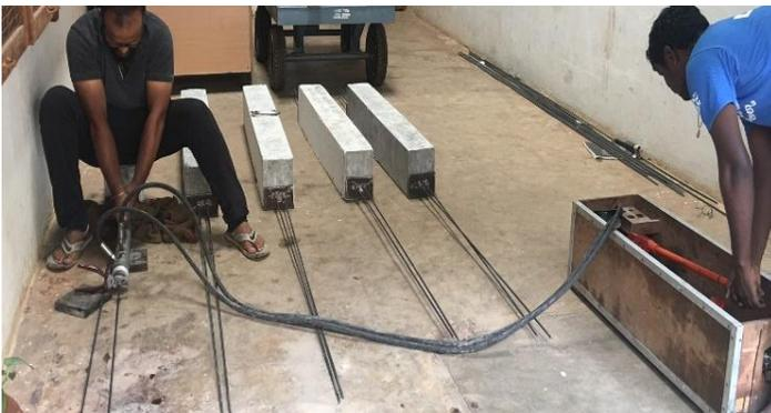
Figure.1. Post-tensioning of beams
