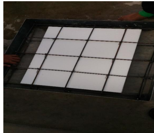
Figure.4. polystyrene tied between reinforcement bars
