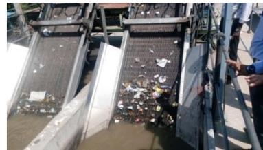
Figure.2. Showing automated screening (captured from the site)
