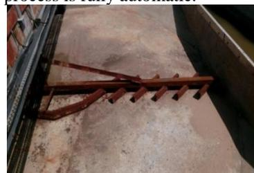
Figure.3. Showing the inner view of grit removal (captured from the site)
