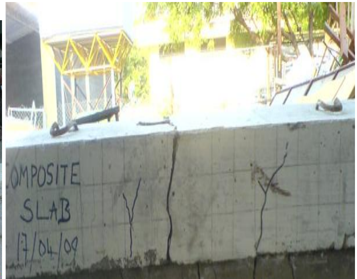
5.4 Composite slab after Testing
