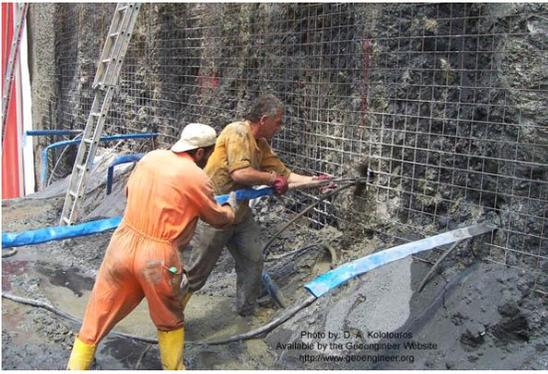
Figure.4. Grout is being placed with the help of pipes
