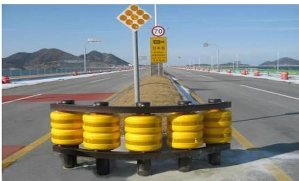
Figure.1. Rolling barrier
