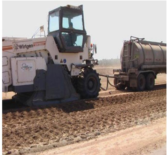
**Figure.2. Mixing of soil-cement for sub-grade stabilization**
