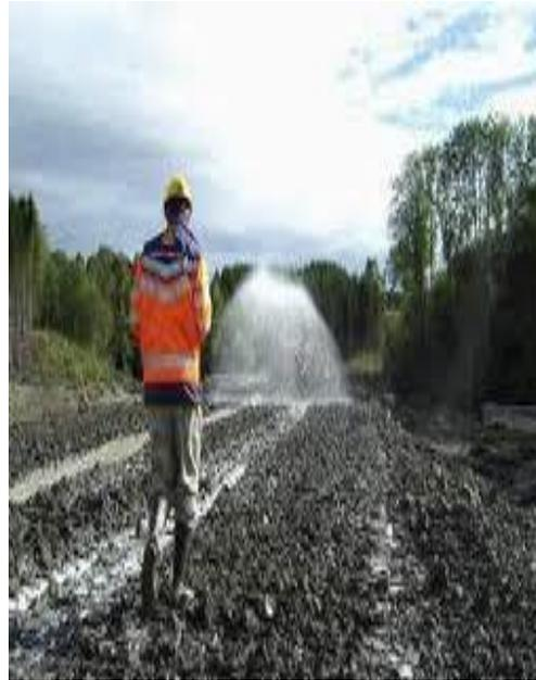
**Figure.3. Soil stabilization with bitumen**
