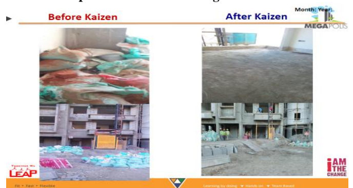
Figure.5. Before & After (Proper Placing of Materials)
