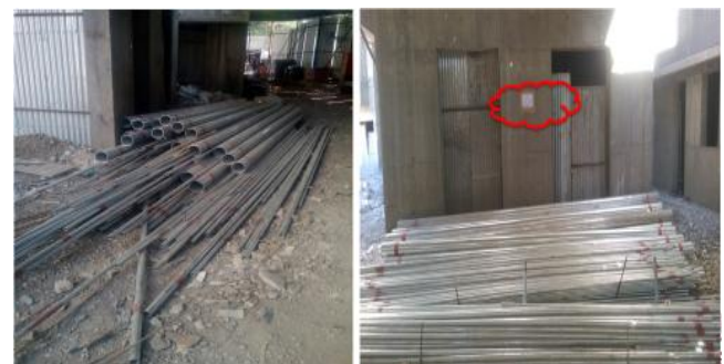
Figure.4. Before & After (Systematic arrangement of reinforcements)
