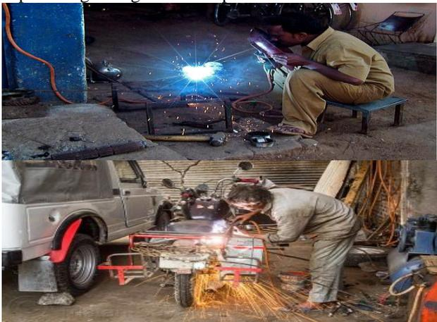
**Figure 4.2 Workers Working Without Proper PPE**
